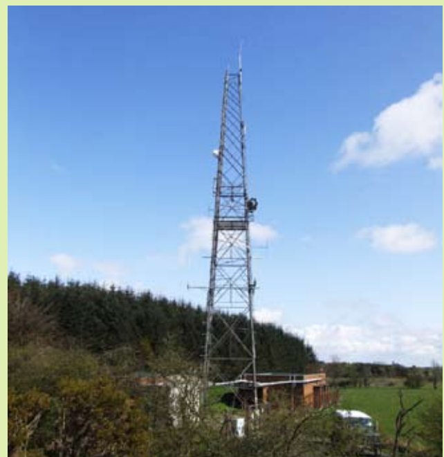
■ One of the two Beacon Ring transmitter masts. Photo CPAT 2561-0046
